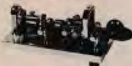
In 1890 Horace Martin searched for relief from the "glass arm" wireless operators were getting from pounding straight keys. He innovated by placing the key on its side and our semi-automatic key was born. Press the thumb piece and the vibrating lever bar produces dots. Make dashes manually with the finger piece. Speeds as low as 20 wpm or as high as practical can be sent with the speed lever. The original bug is still buzzing wherever speed and perfection are desired.
