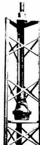
Top section of a Ham Tower with a rotator, mast and a Model BBMB installed.
