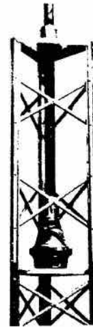
Top section of a Ham Tower with a rotor, mast and a Model BBMB installed.
