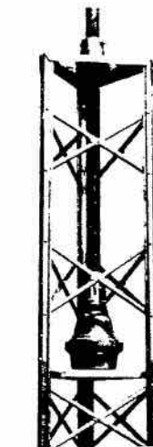
Top section of a Ham Tower with a rotor, mast and a Model BBMB installed.
