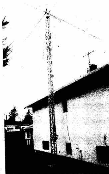
10. Tower complete with antenna.
