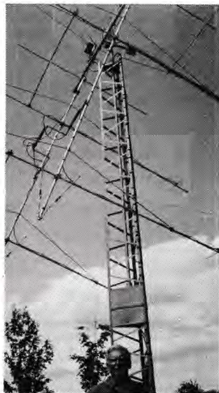
"The Bird", Ted Sparrow, VE3BQN, and his 2-metre EME array. Eight Cushcraft Boomers put out a big signal from Elmvale, Ontario. (VE3CDM photo)
