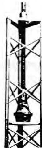
Top section of a Ham Tower with a rotator, mast and a Model BBMB installed.
