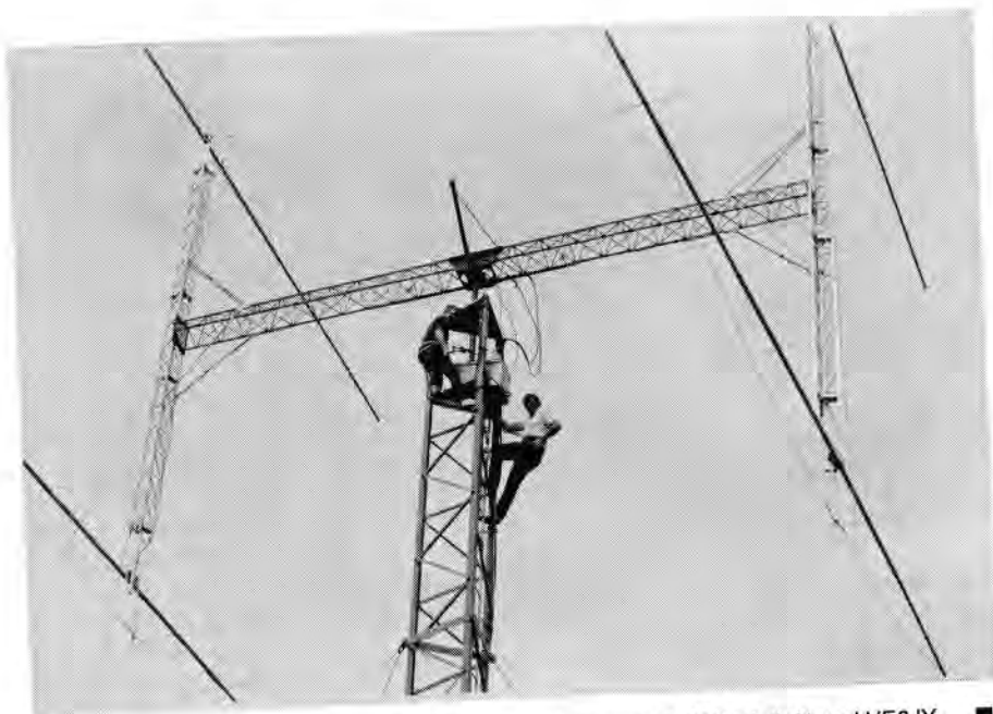
Six-metre EME array at VE6JW/VE6EME. Up on "the beast": VE6MAA (left) and VE6JY. ■
