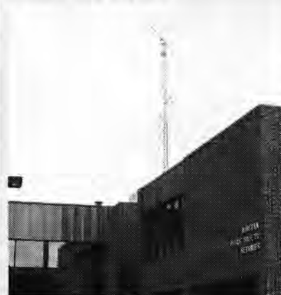
The VE6GOC HF and VHF antennas tower above the Edmonton Headquarters building of Alberta Public Safety Services. A good looking setup! (Photo courtesy VE6BLY)
