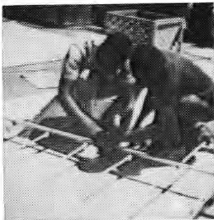
Assembling the 2-metre beam: 40 metres might have worked better.
