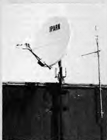
The Inter-Provincial Amateur Radi Network (IPARN) Ontario earth station with UHF Yagi for links to local terrestrial networks. (VE3NGT photo)
