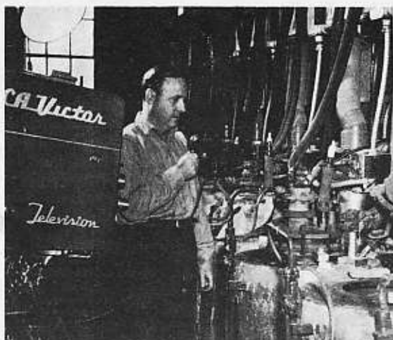
An RCA TV camera makes it possible for stockholders to witness the complex processing of rare elements at the Foote Chemical plant.
