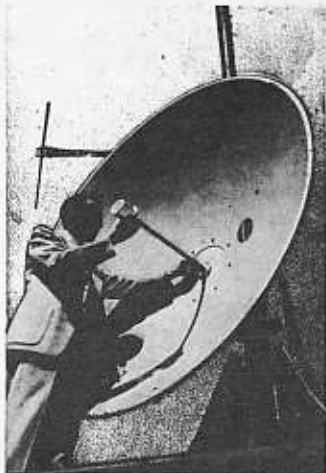
One of the 114 communications system microwave reflectors for the Transcontinental Pipe Line Corp., to extend over 1840-mile pipe line under construction between Houston and New York.
