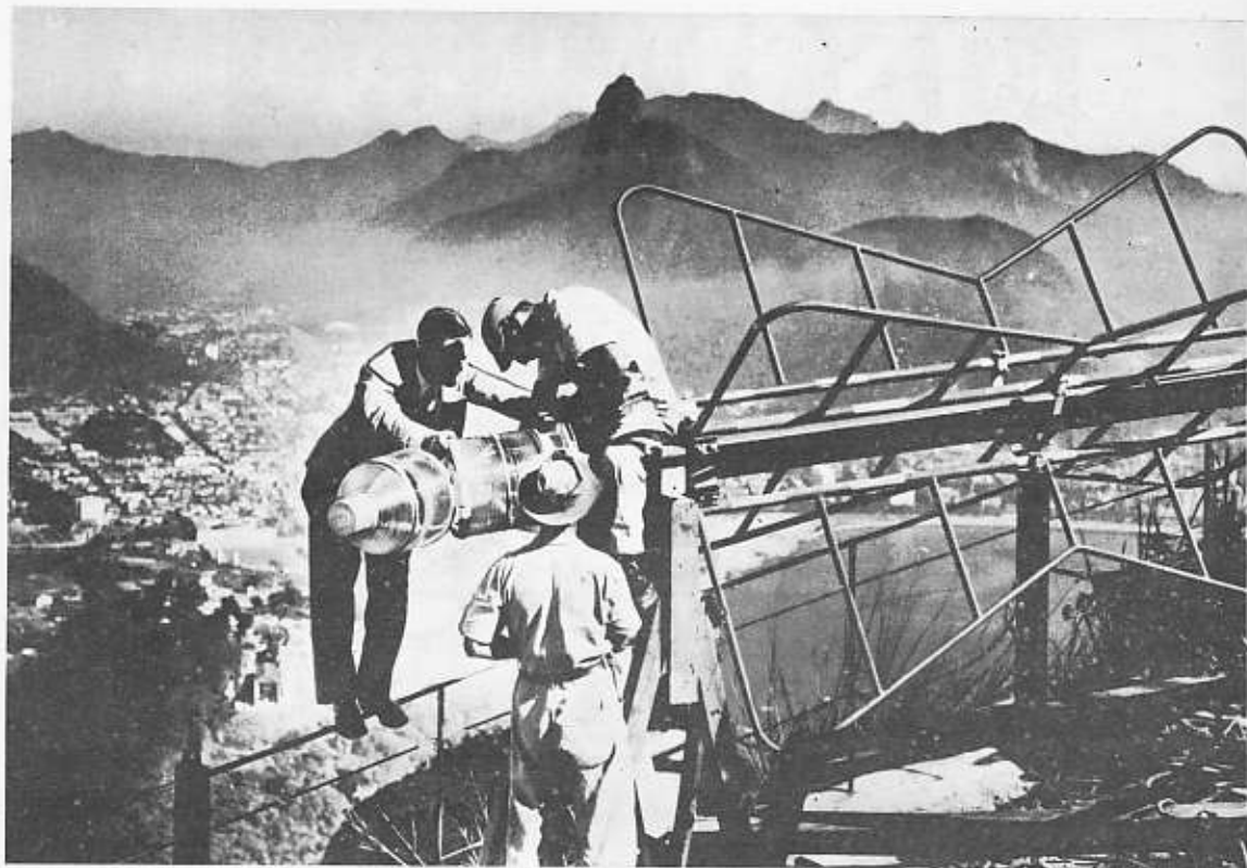
To give Rio de Janeiro its first television programs, engineers of the International General Electric Company installed transmitting equipment atop famed Sugar Loaf Mountain high over nearby Copacabana Beach. Several tons of equipment, including the 150-foot antenna, had to be hauled by cable car, mule-back, and by hand to the mountain summit.
