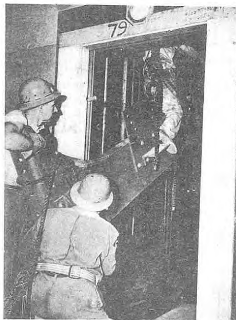
Steelwork for the 217-foot tower is raised from ground level to the top through one of the building's elevator shafts.
