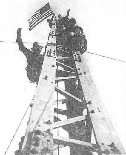
Intrepid riggers hail the completion of the lofty structure by raising a flag on the tower's peak, 1500 feet above the street.
