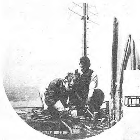
Workmen with torch and sledge prepare to dismantle the old antenna mast which supported WNBT's TV radiator.
