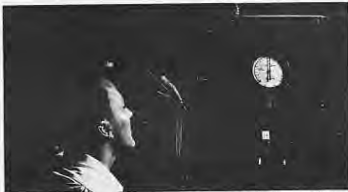
Screens through which seawater enters the laboratory tend to become clogged with seaweed. This instrument, devised by test engineer Dick Bradshaw (above), tells when it's time to have the screens cleaned.
