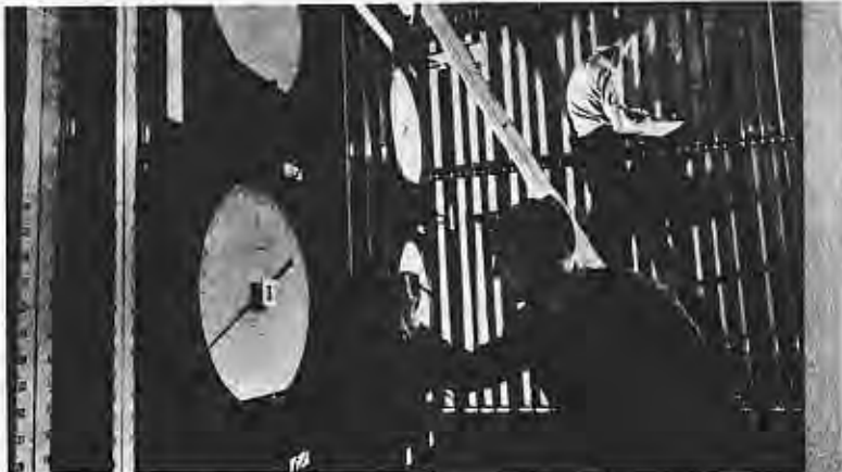
Hundreds of instruments like these record the progress of research tests on engine parts in the new lab. From a main control room an engineer directs operations by means of an intercommunication system.
