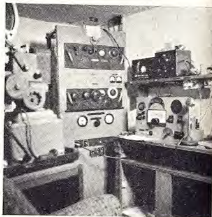
Ve3AEL's rig gives forth with 10 meter fone sigs. Is in projection booth as may be noted at extreme left.
